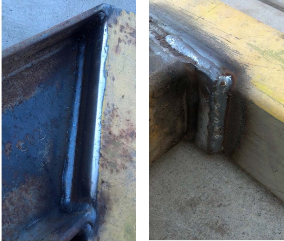
Figure 17. Finish welds.
