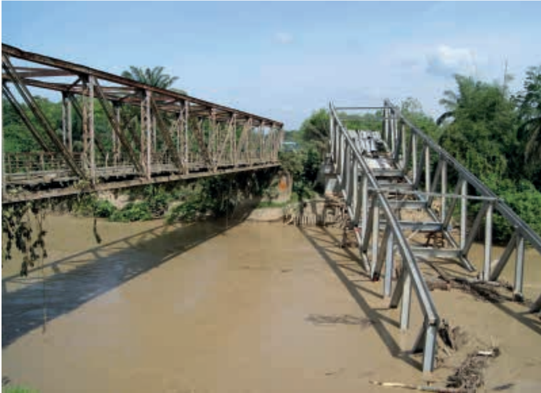
The route to market can be difficult. The bridge built by the Dutch many years ago is still standing, although it takes a little nerve to travel over it as the rotting beams crack and creak under a vehicle. The replacement bridge built by the Indonesian engineers is not quite so able to cope with the regular earthquakes and river flooding. Saggaf told us that this was the third time it had fallen into the river since it was built.
