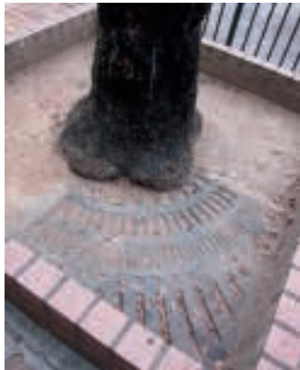
Badly designed tree pits filled with very compacted soil and concrete, with poor maintenance.
